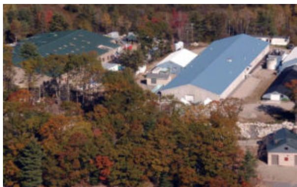
USDA (left) and University of Maine research buildings during construction in the fall of 2006.
