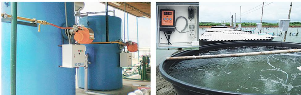
Gas-powered heaters (left) provide warm water to raceways in a Peruvian shrimp farm. Electric heaters maintain water at  $32 \pm 1$  degrees C to control WSSV at a Thai farm (right).
