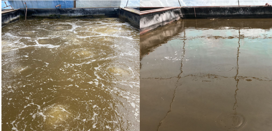
View of tanks with an activated aeration system (left) and without an aeration system (right).
