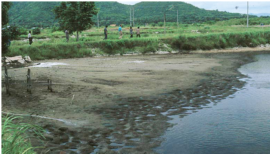
Sedimentation pond showing accumulation of solids at water entry point at left.
