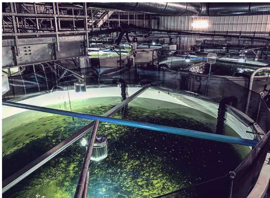
An indoor view of the Atlantic Sapphire Bluehouse™ outside of Miami, Fla. Photo courtesy of Atlantic Sapphire.
