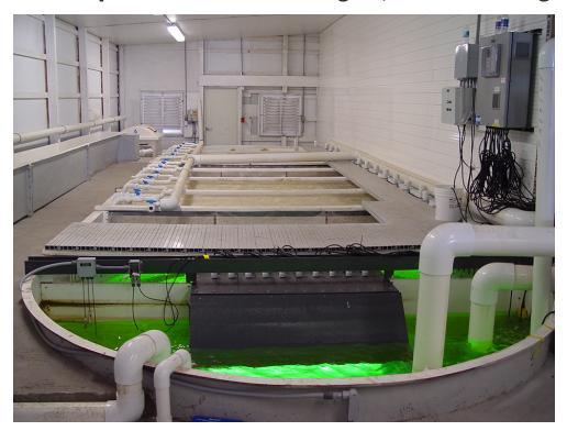
Even if a facility has a properly sized or even oversized biofilter, as in this large moving-bed biofilter with ultraviolet treatment, yet the flow between the biofilter and culture tank is too slow, the biofilter capacity will never be fully utilized, and ammonia nitrogen can build up in the culture system. Photo courtesy of Mote Marine Lab.
