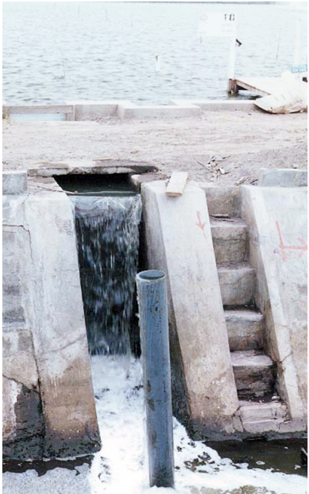
Settling basins are the only practical means of treating pond effluents (above).
