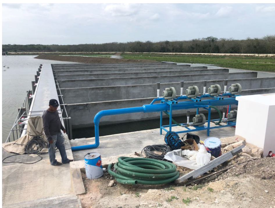
View of the raceways used in this study (background) and the bank of blowers (foreground) that support strong water flow and aeration inside the IPRS units.
