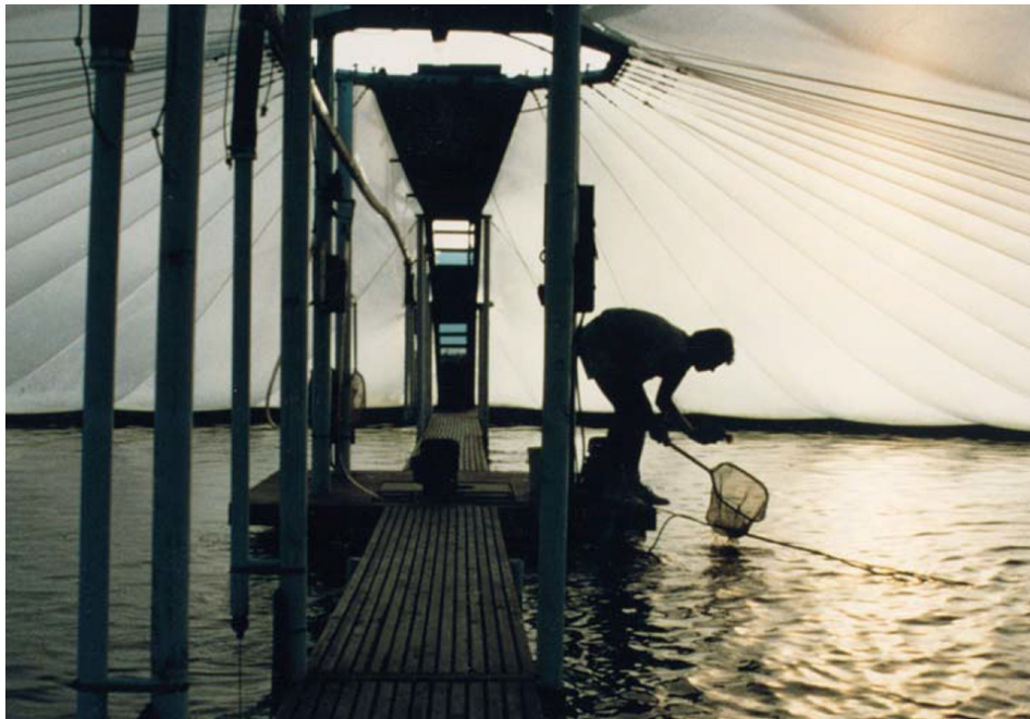
Fig. 2. An inside view of grow-out tanks in the Solar Aquadome. The 96-foot diameter tanks are covered by tensile structure greenhouses.
