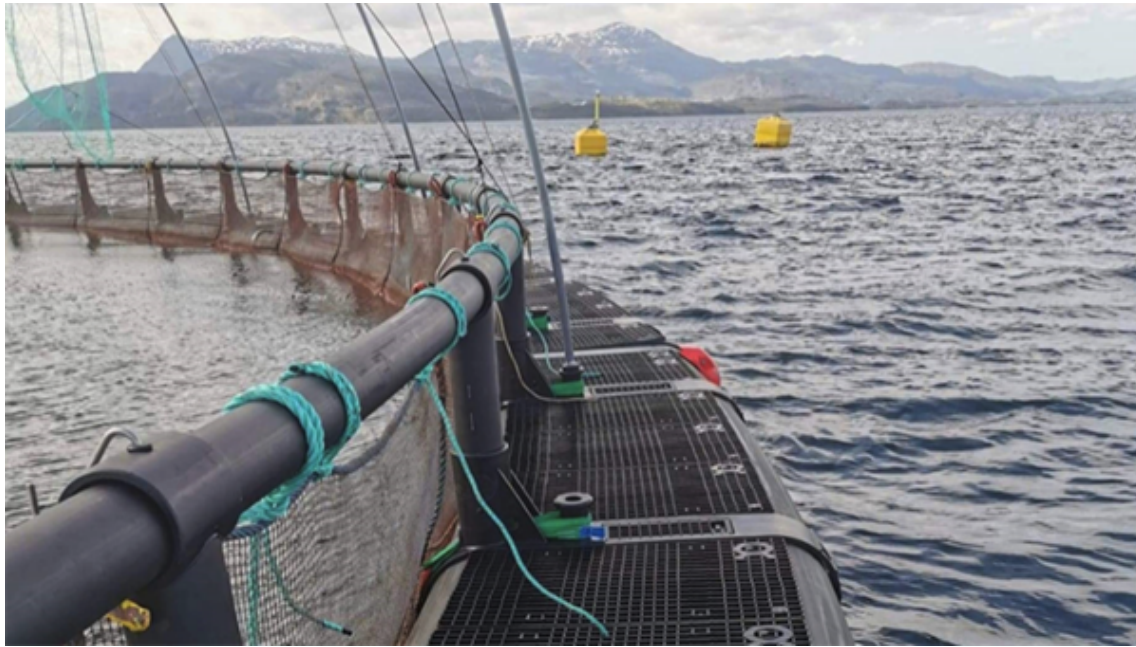
An ocean net pen built without polystyrene. Photo courtesy of AKVA Group.
